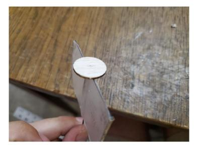
Attach a gusset between the disk and the carbon rod.
